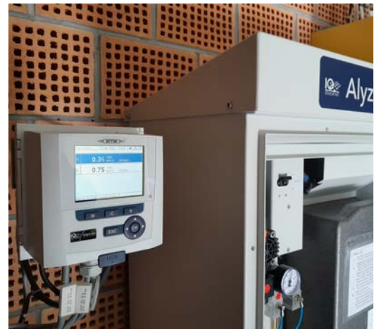
Figure 2: Alyza IQ \text{NH}_4 (2-channel) connected to an IQ SENSOR NET controller DIQ/S 282-CR3
